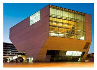
which develops the mandatory spaces of the program. The envelope is made of concrete with slopes that reach 48°. The building was a constructive challenge. It took 12 months to study how to "get it" to build. Its construction was carried out in 85 phases, each with its stability calculation.
